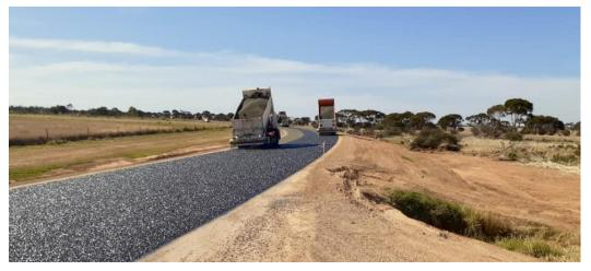
The completion of capital roadworks along Ferguson and White Streets, spanning from Maddock to Shadbolt Street, marked a significant achievement. This comprehensive project encompassed various enhancements, including 2x 2.5-meter edge reconstructions, kerb replacements, and a full 7mm single coat reseal covering the entire road surface from kerb to kerb.
