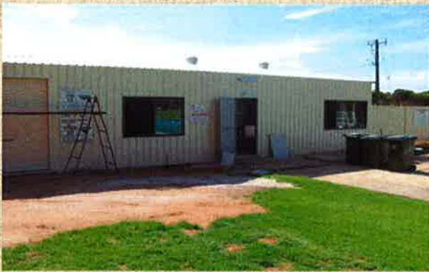
Swimming Pool Upgrade Stage 1 New Pump Shed
