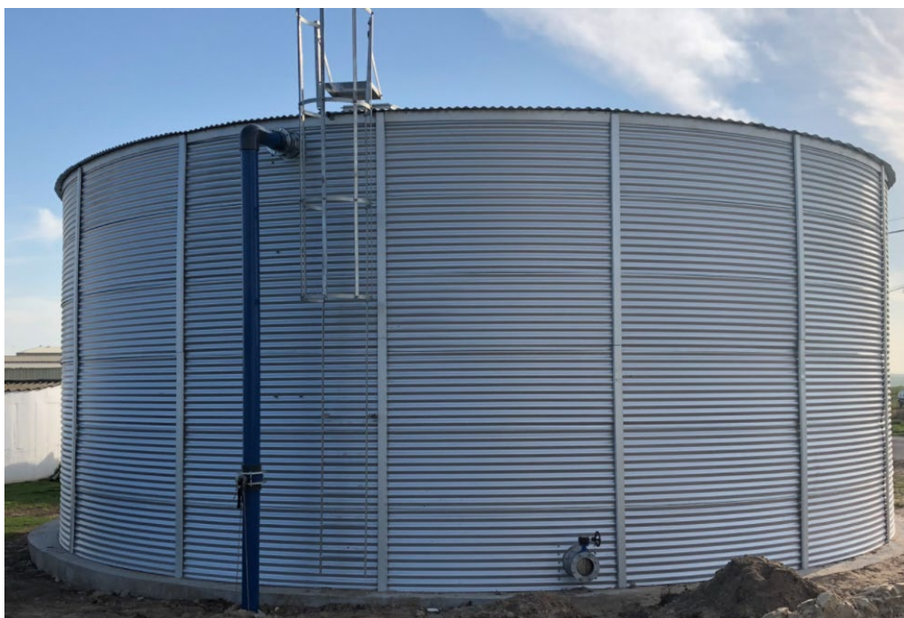
Above: 360,000ltr metal tank.
