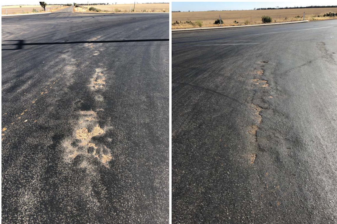
Above: Exposed gravel at the intersection and bad flushing pre-sealing.
