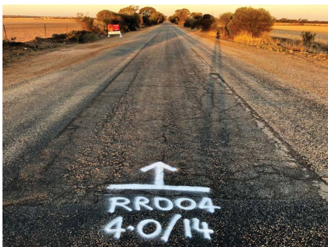
Above: Wilgoyne Road immediately east of Mukinbudin Wialki Road, bad cracking and potholes obvious.
