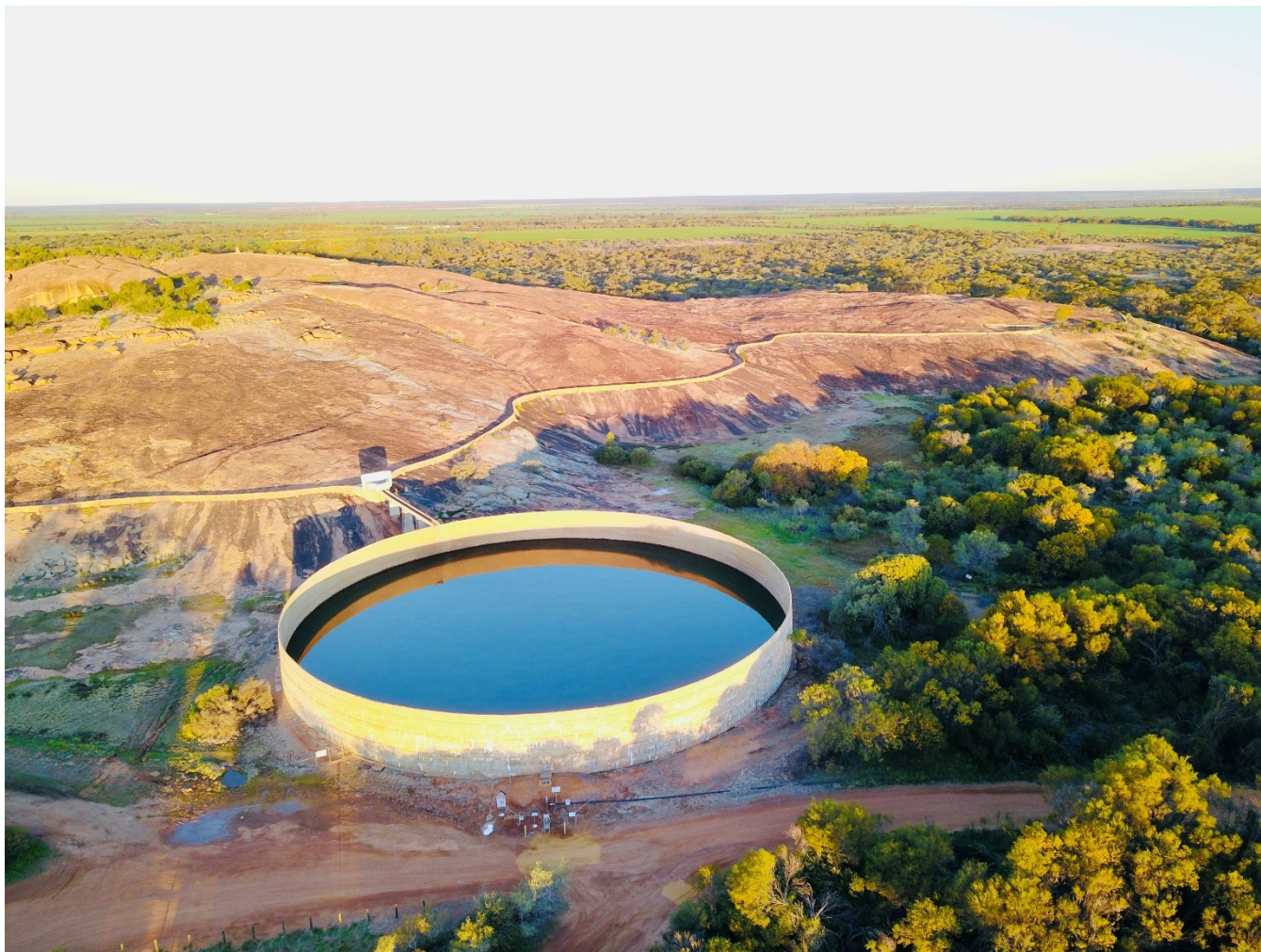
Above: Beringbooding Tank after roof removal – August 2021
