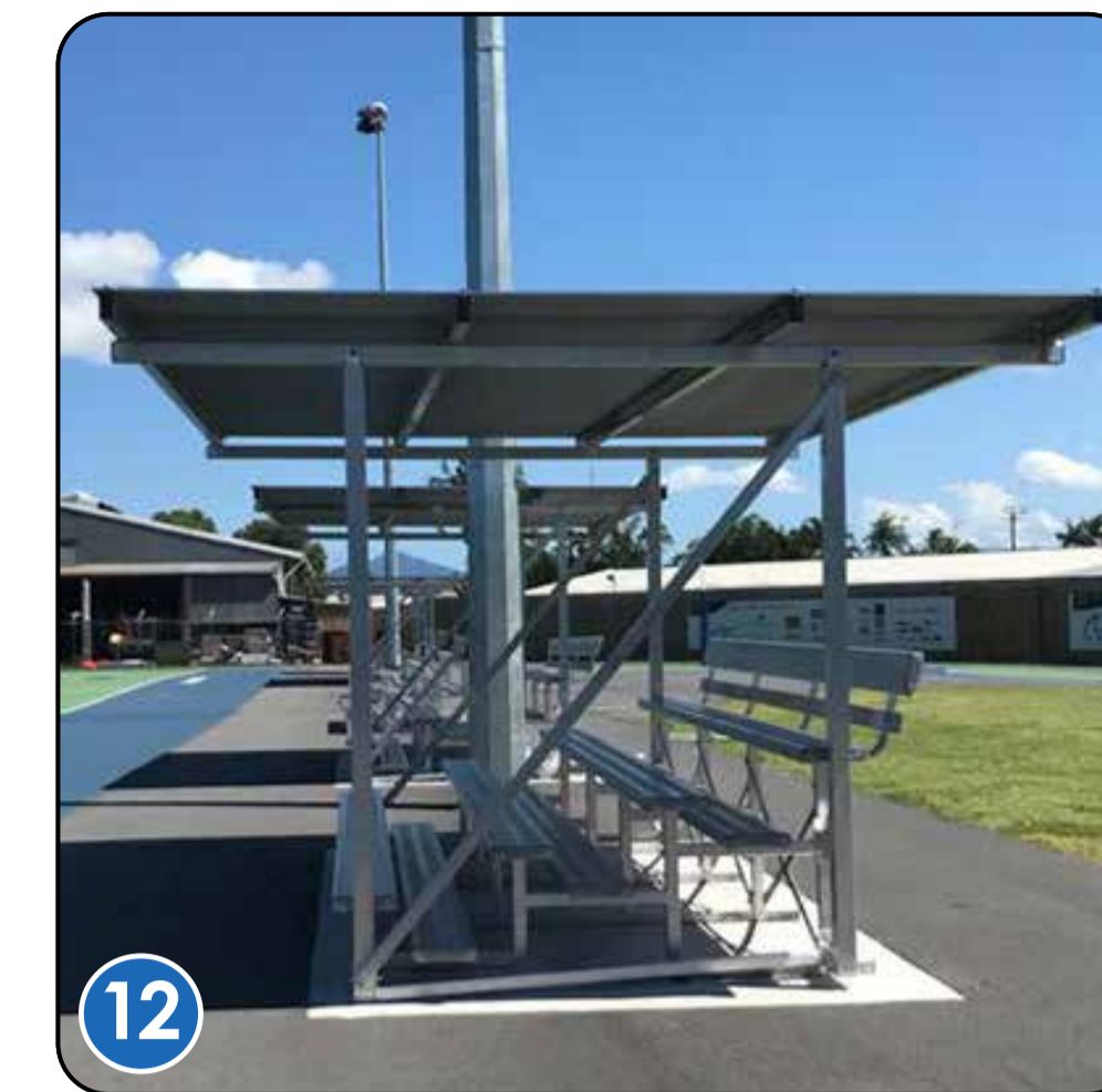
12 Bleacher grandstand seating. Two set up back to back for dual use with tennis court and pump track viewing. Grandstand by Felton Industries.
