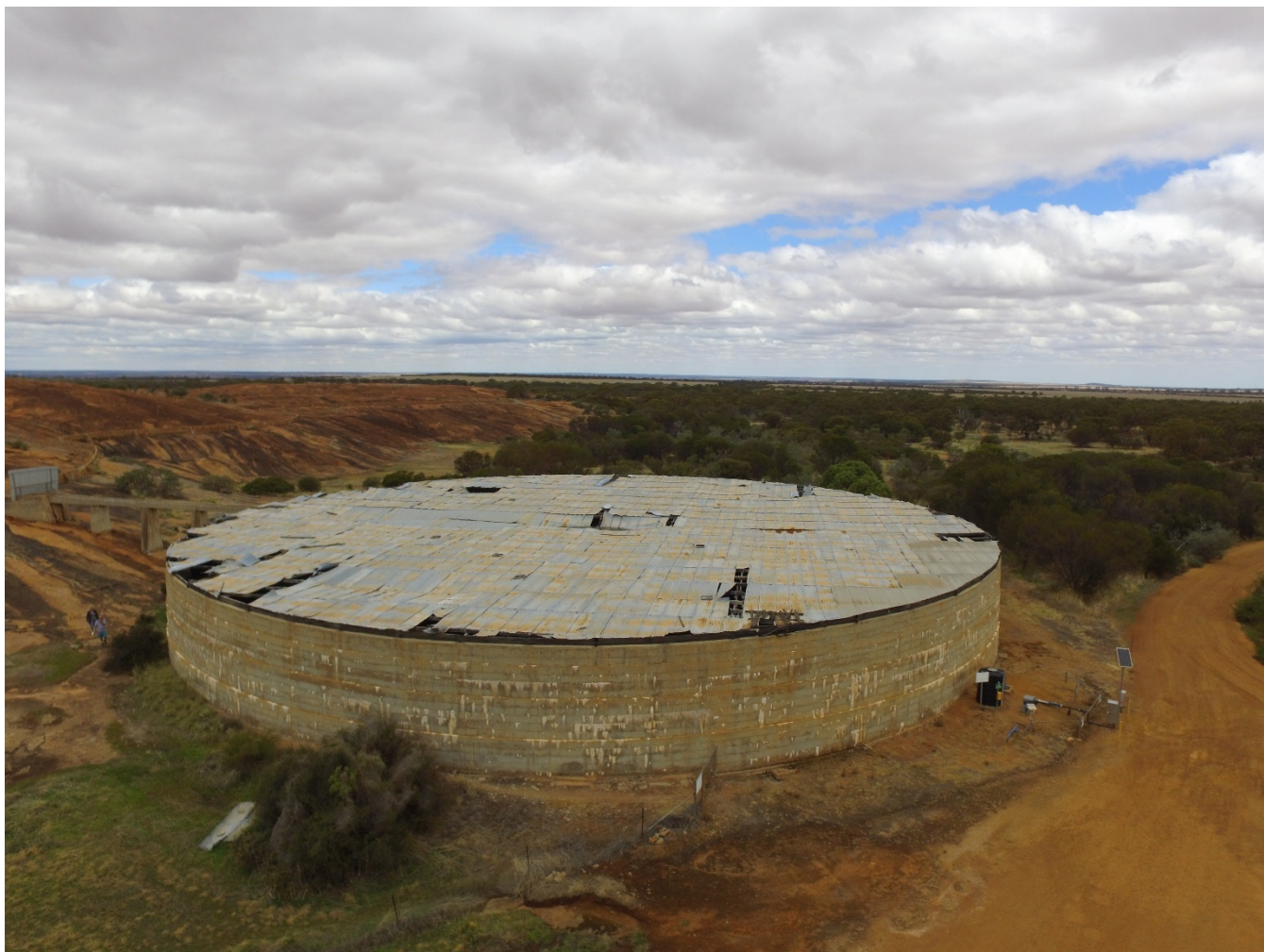
Above: Beringbooding Tanks Roof – July 2018
