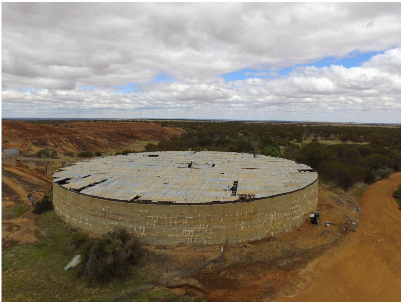
Above: Beringbooding Tanks Roof – July 2018
