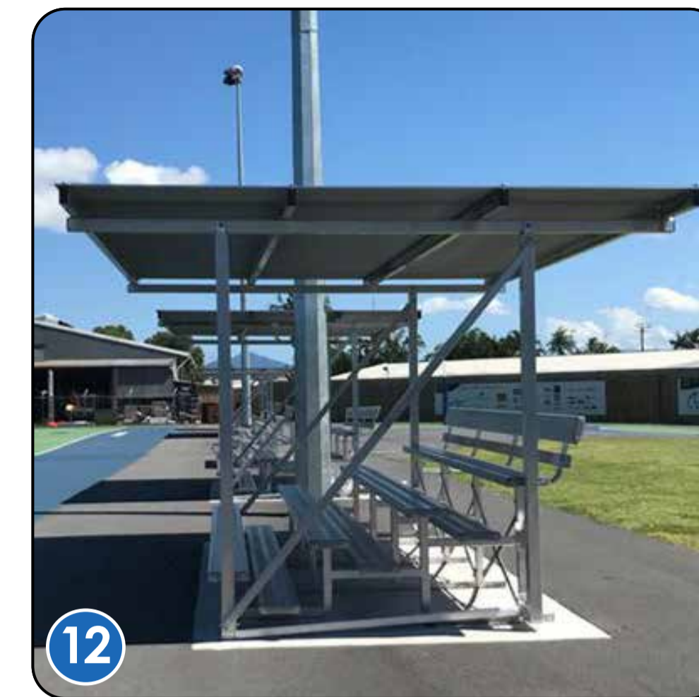
12 Bleacher grandstand seating. Two set up back to back for dual use with tennis court and pump track viewing. Grandstand by Felton Industries.
