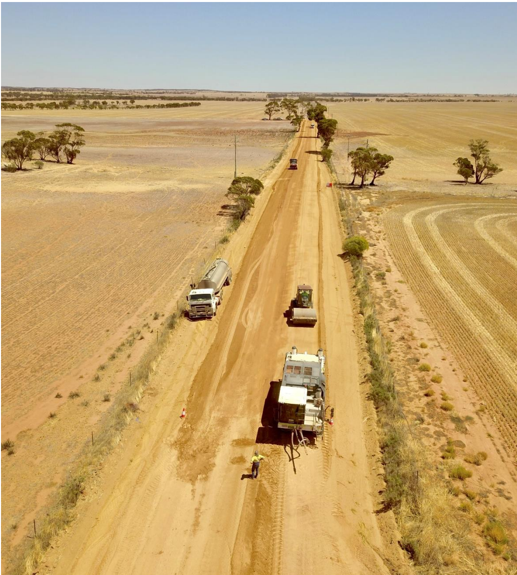
Wet mixing of Kununoppin Mukinbudin Road March 2022
