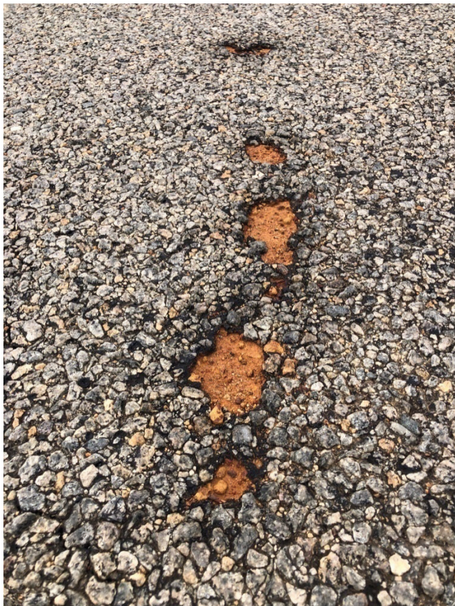
Above: Nungarin North Road bitumen fail
