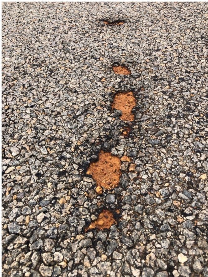
Above: Nungarin North Road bitumen fail
