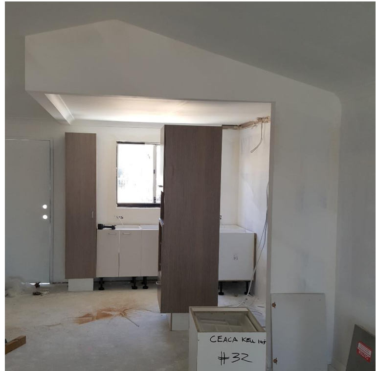
Cabinetry works in a kitchen area
