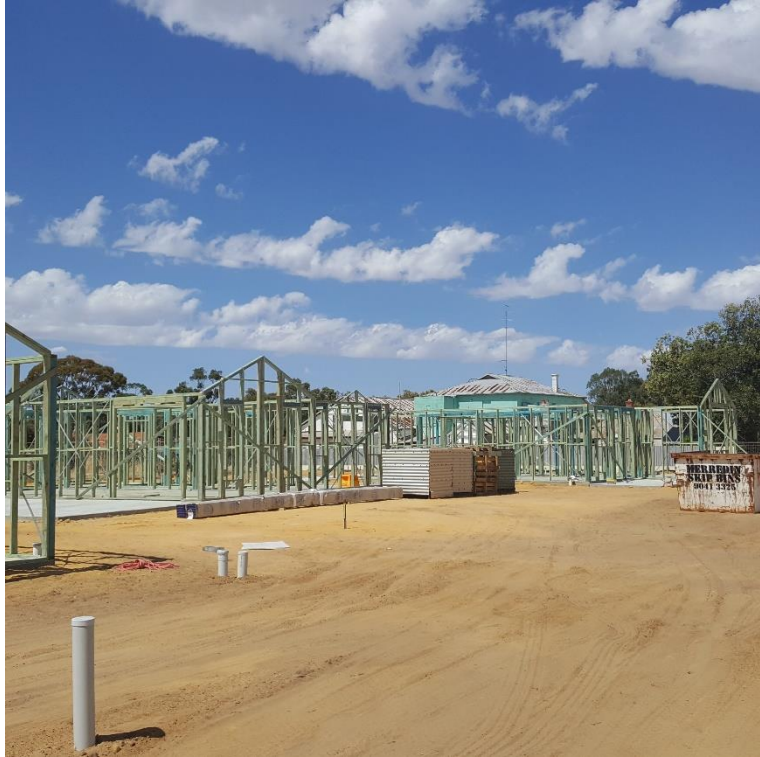
Framing commenced at Bruce Rock
