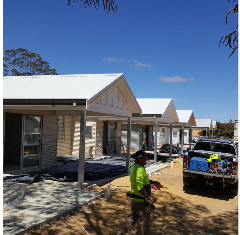
Kellerberrin units at lock up stage
