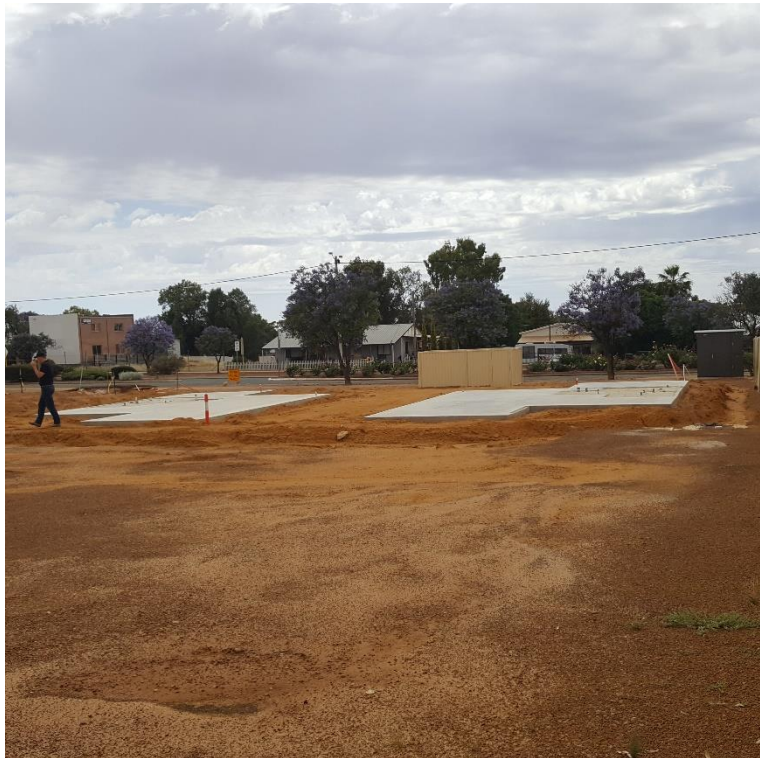
Slabs down at Yilgarn
