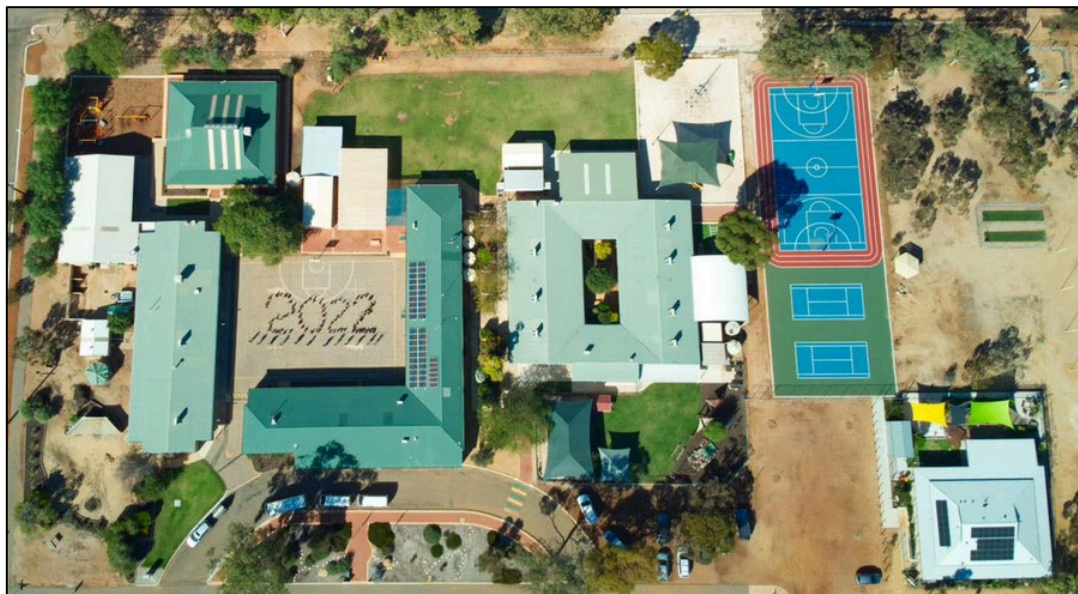
Above: Aerial photograph of the Mukinbudin District High School.
