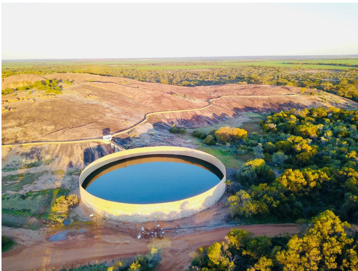
Above: Beringbooding Tank post roof removal circa July 2022
