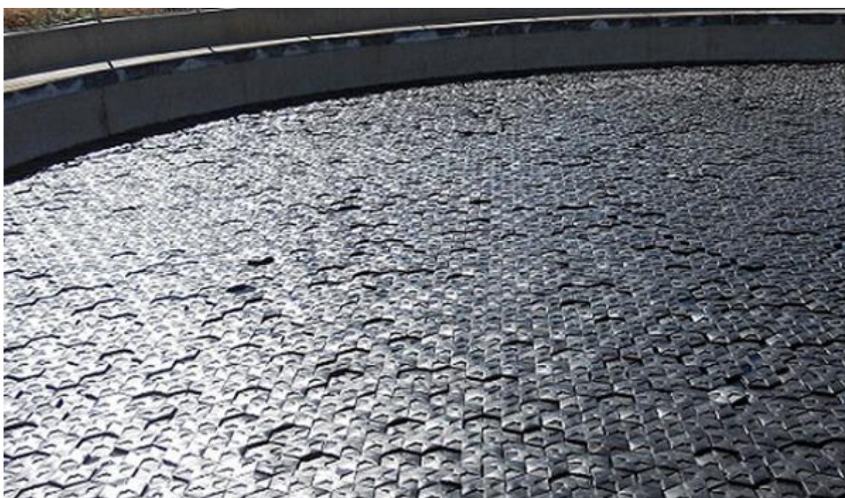
Above: HexaCovers floats in a large water tank, southern Western Australia.
